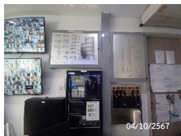
Graphic Annunciator Fire Alarm System
